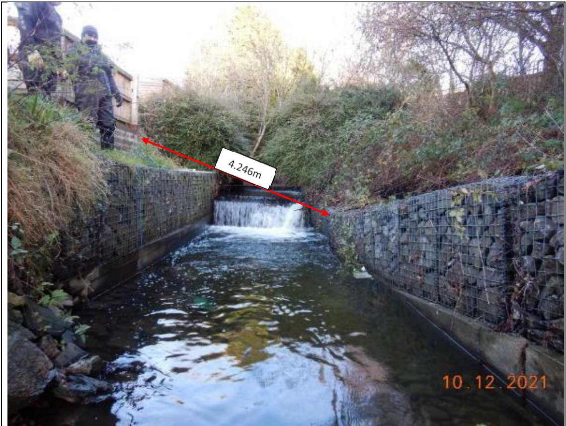
Distance from Block Wall to Gabion opposite
