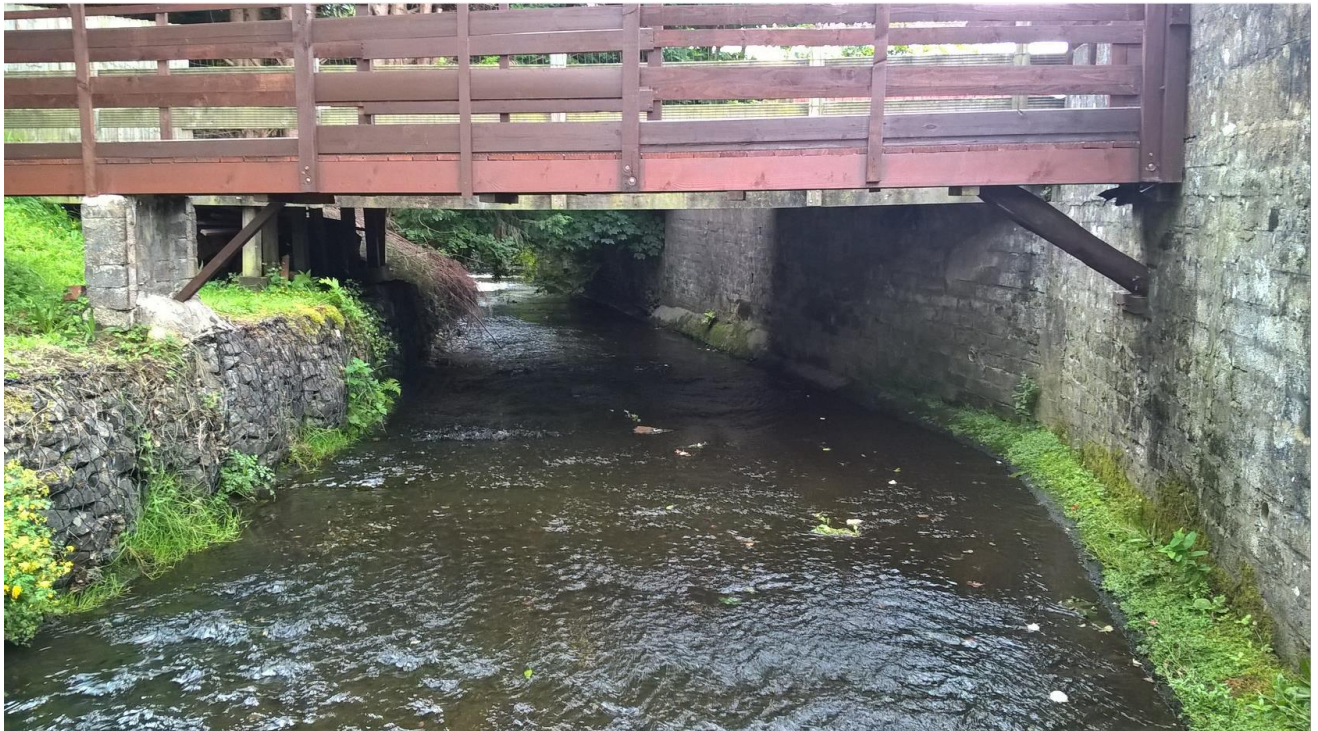
Figure 2 – Section 1: Concrete lined channel and bank retaining structures
