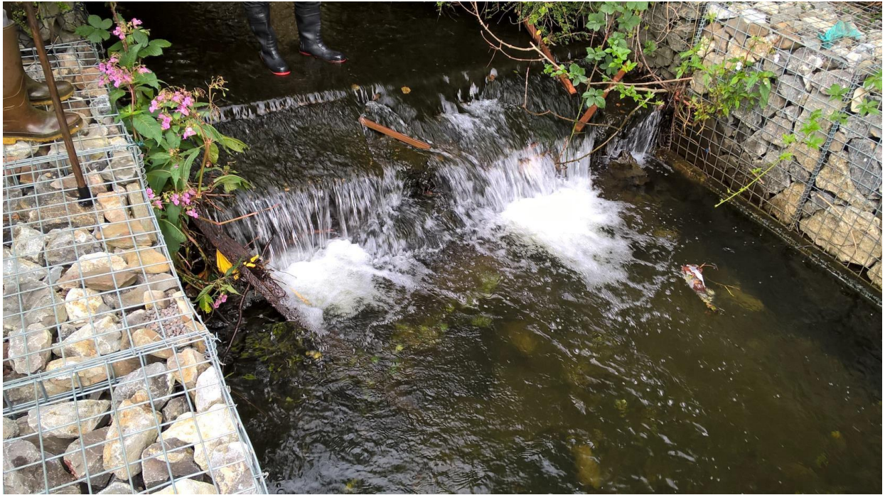
Figure 3 – Section 2: Concrete weir
